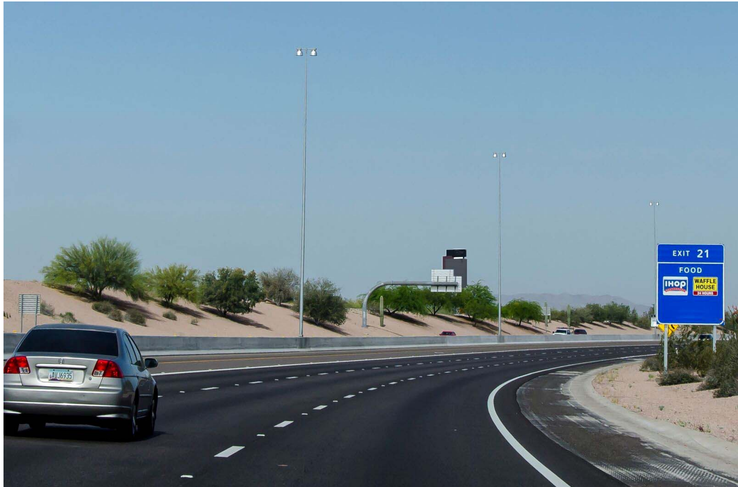
Sign 2: 50ft. Westbound Just Past Higley On-ramp
