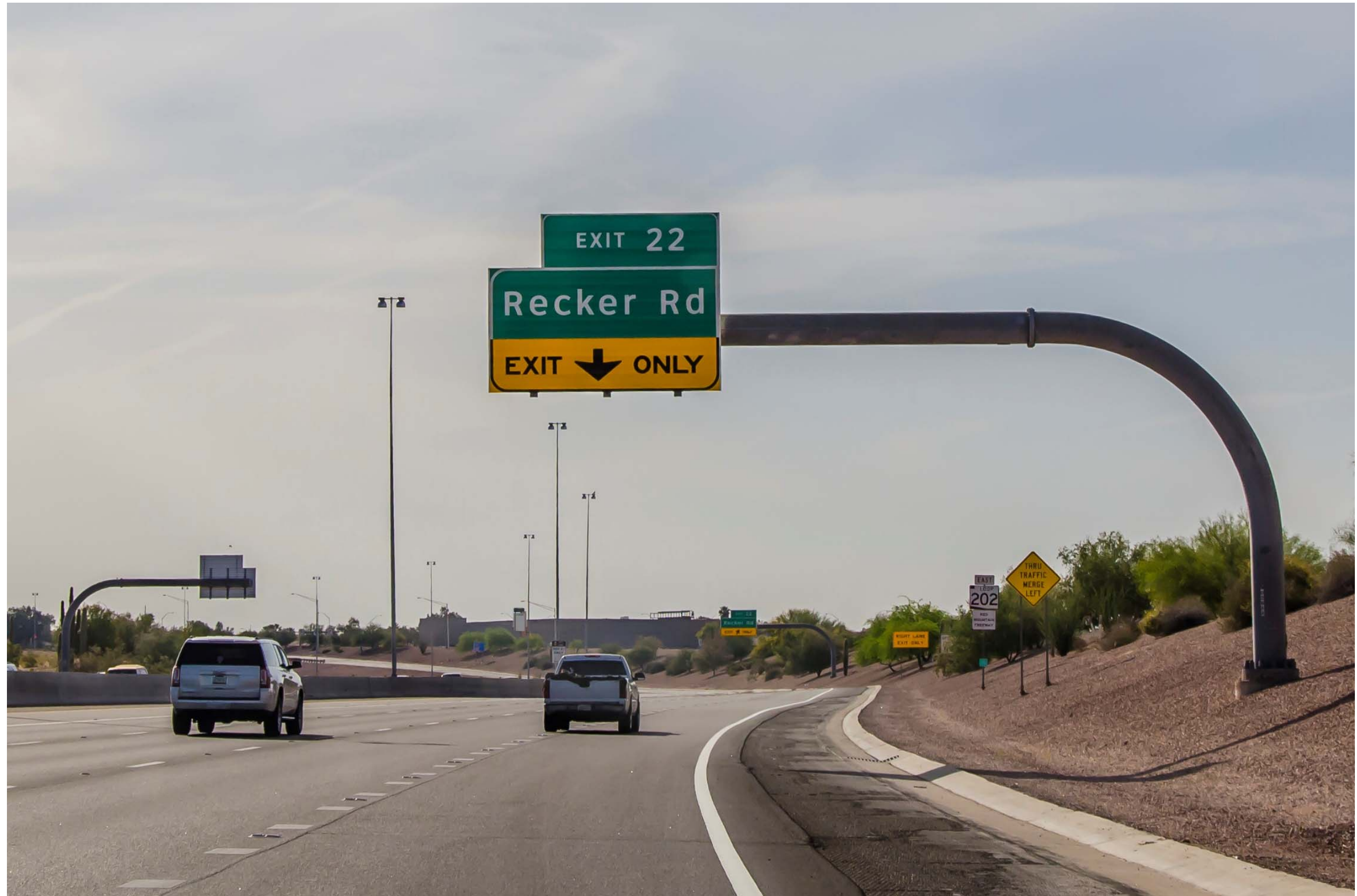
Sign 1: 40ft. Eastbound Towards Recker
