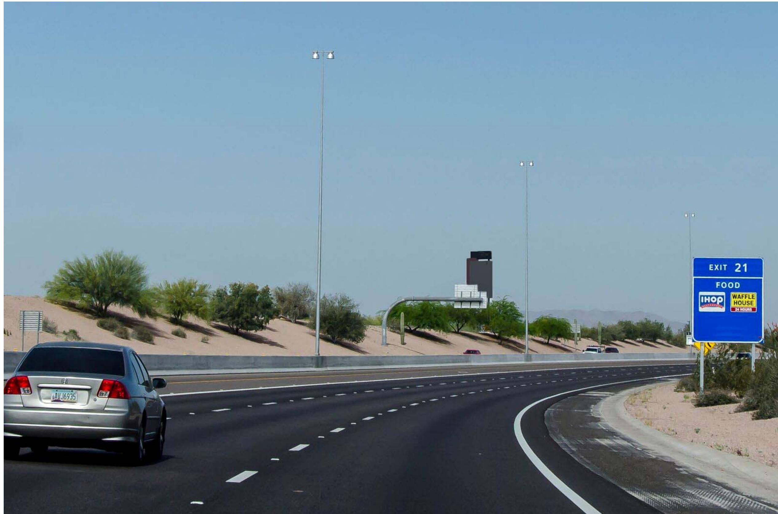
Sign 2: 60ft. Westbound Just Past Higley On-ramp
