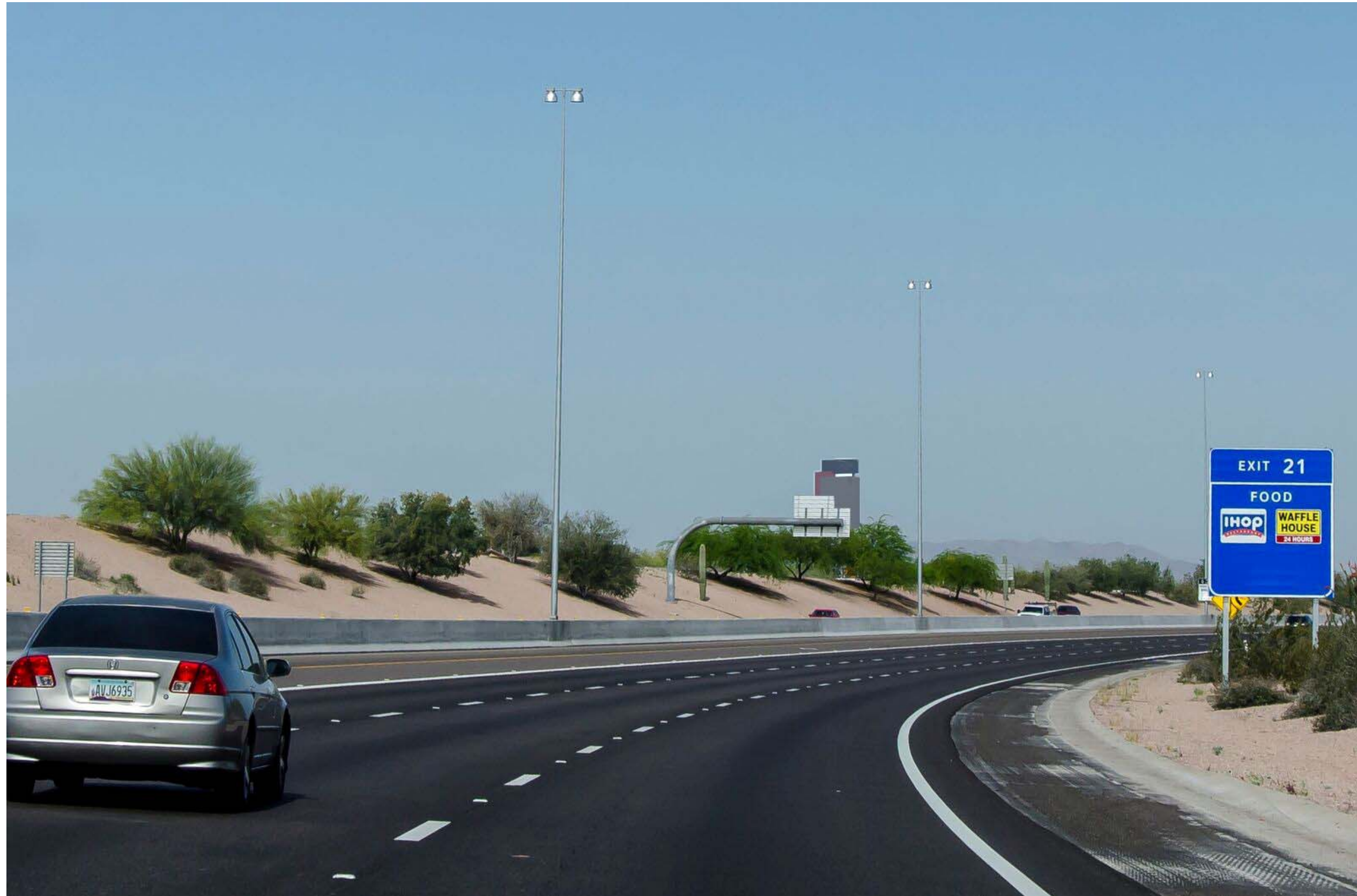
Sign 2: 40ft. Westbound Just Past Higley On-ramp
